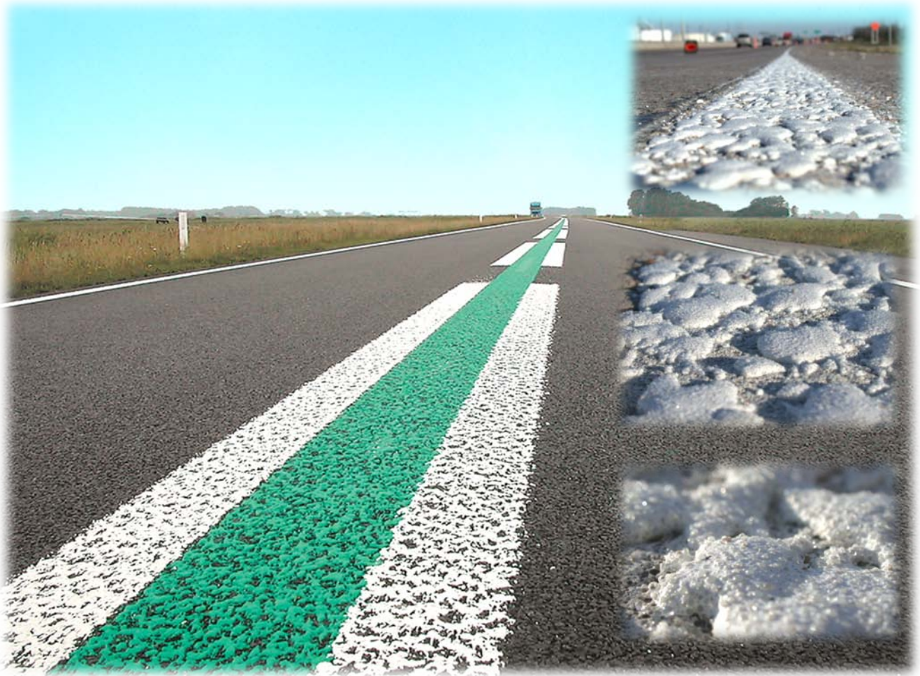
Stochastic agglomerate markings with scattering drum
