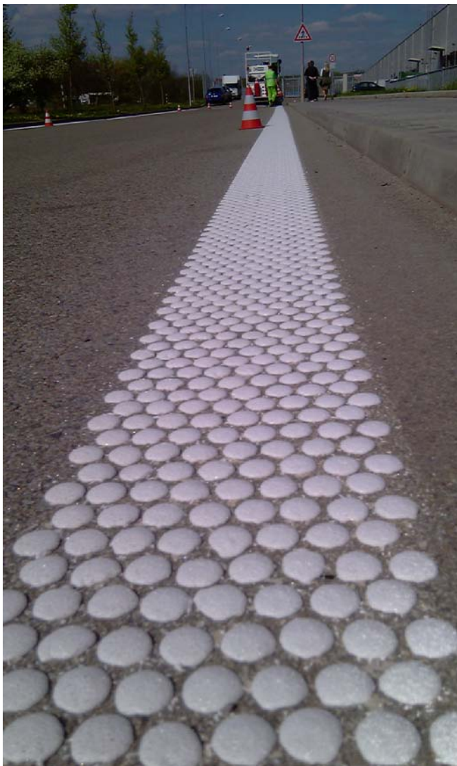
Figure 5 2-component cold plastic SPOTFLEX ® roadmarking
